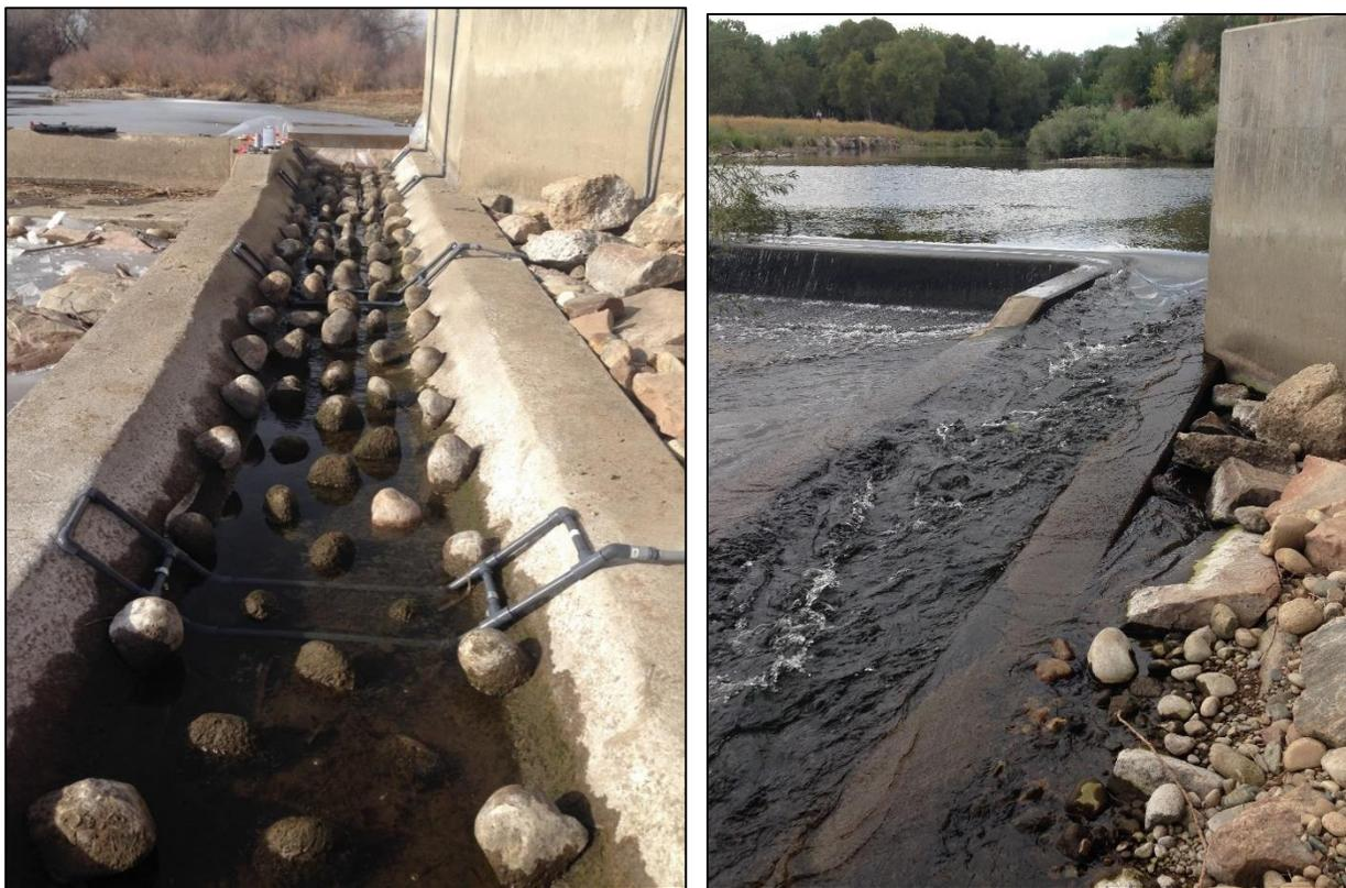
**Figure 2.3-** The Fossil Creek Reservoir Irrigation Diversion (FCRID) site in Fort Collins, CO, USA, with the left photo (A) showing the antenna placement on the interior of the rock ramp and the right photo (B) showing the fishway during moderate flows.
