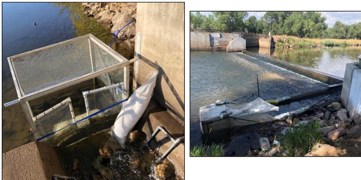
**Figure 2.4-** Images showing the installation of the top (at left) and bottom (at right) enclosure boxes for the trial at the FCRID site.
